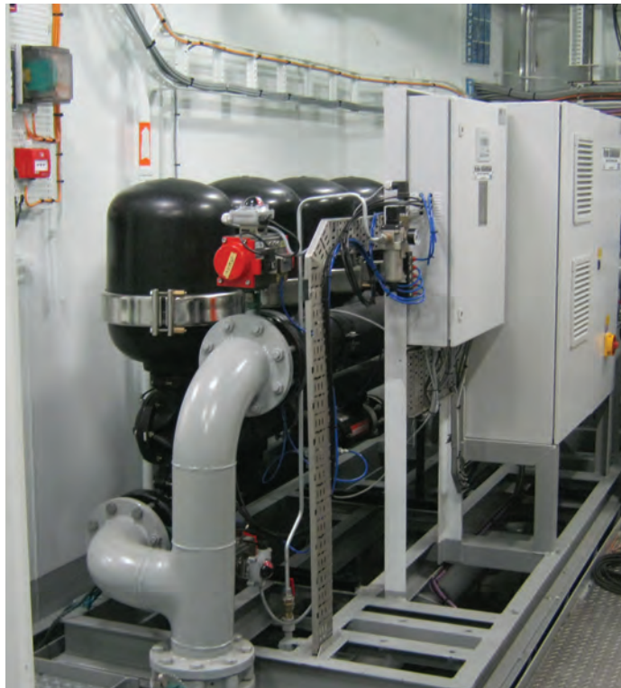
HG150 pictured on board New Construction Offshore Service Vessel
