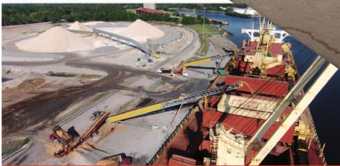
ONE MACHINE LOADS, TRANSFERS AND STOCKPILES
