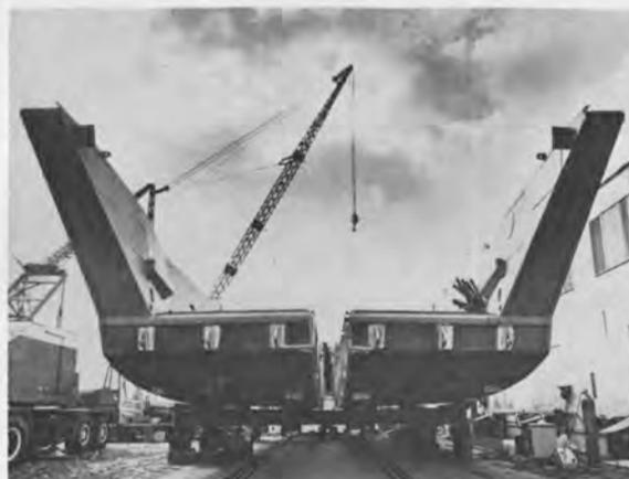
At San Diego—When the two sections of the landing craft are aligned, they are welded together by pairs of welders, starting at the craft's center and progressing at the same rate in opposite directions. New shielded aluminum arc-welding equipment insures excellent penetration at rapid welding rates.
