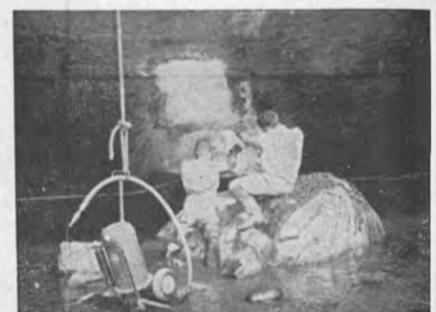
Damaged Liberty hull was sealed with CORDOBOND resins and fibre glass prior to refloating—Costly gas freeing was eliminated.
