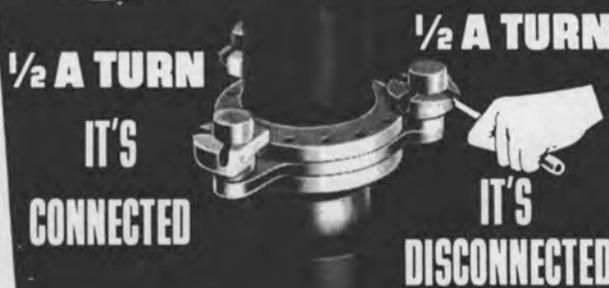
Quick acting cams do the "trick". Less than one turn sets each cam and locks the O-Ring gasket forming a leak proof seal. Drastically reduces operating costs.
