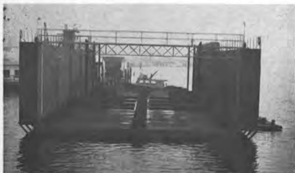
**NEW FLOATING DRYDOCK** put into operation by Martinolich Shipbuilding Corporation, Tacoma, Wash. The 1,250-ton lifting-capacity dock is provided with four centering posts controlled from the control tower, enabling the dockmaster to center the vessel quickly. The bilge blocks are attached to the centering posts and are cranked in from the vessel instead of the wingwall. The drydock is new in every respect and has been certificated by Philip F. Spaulding & Associates, Inc., of Seattle.
