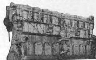
Type LS—15 1/2 x 22—turbo-charged engine—BHP 1300 @ 270 RPM. Air starting @ 250 lbs. Complete with air tanks, heat exchanger and all accessories. Preserved in equal-to-new condition. Also spare pistons, cylinder liners, valves, etc. Still aboard Corps of Engineers vessel. Serial No. 2172—Buchi Turbo-charged.
