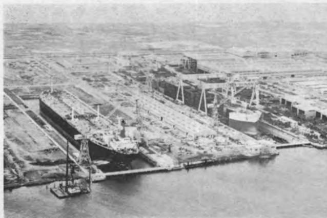
The capacity of our Sakai Shipyard has been vastly increased with the completion last October of a new 400,000 DWT dock. It can easily accommodate the largest ships afloat today. The dock measures 380 meters in length, 62 meters in width and 12.5 meters in depth and is equipped with the latest facilities for ship repair.
