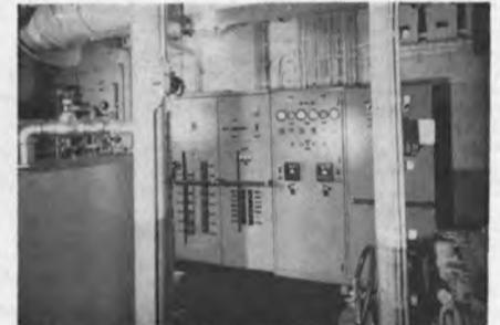
Electrical switchboard contains distribution panel (left), generator panel (center), and capstan control (right).
