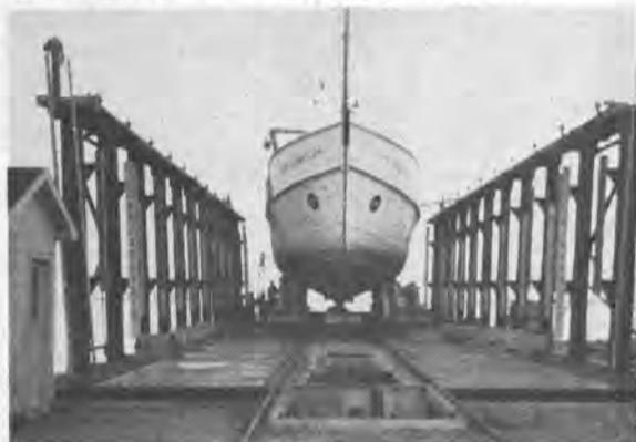
The trawler Jean Cabot was the first vessel to be dry-docked and transferred for winter storage on the new railway dry dock and transfer system at Caraquet.
