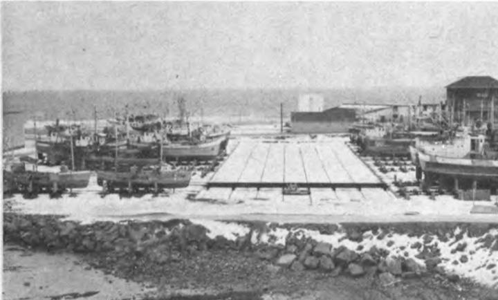
Twenty longitudinal storage berths serviced by a self-propelled cross transfer table.
