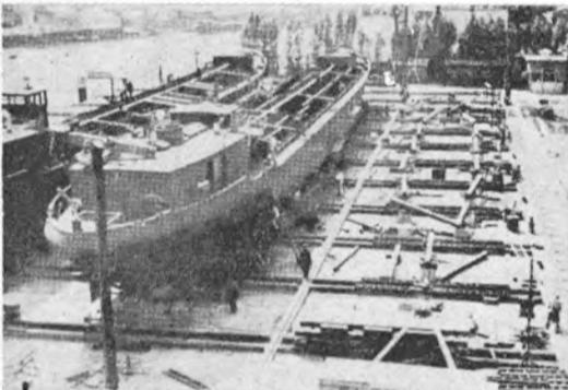
300 ton side transfer system used for barge construction with launching by means of side-haul railway, Dordrecht, Netherlands
