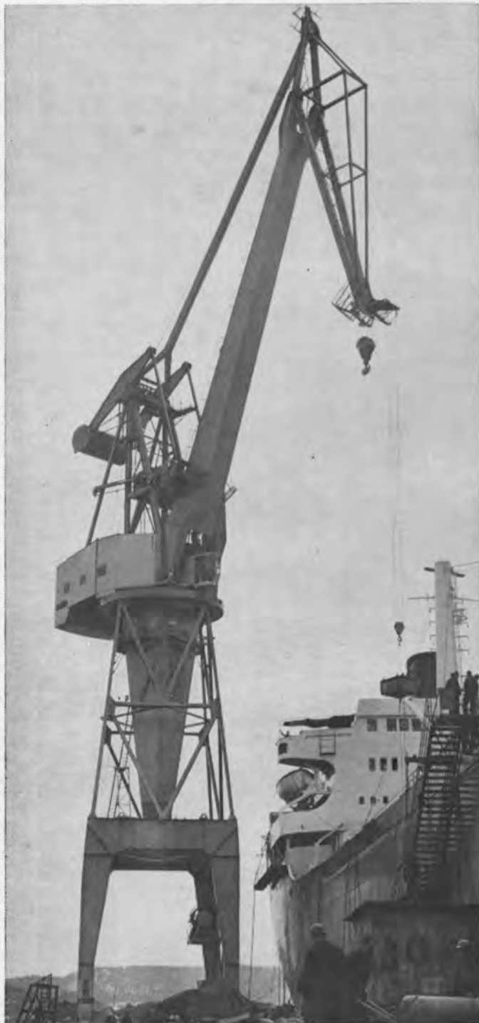
Modern fitting out crane with Ward Leonard stepless electronic control; erected by pontoon method, Capacity: 90 tons/85 ft., 30 tons/175 ft. radius
