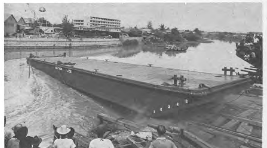
LAUNCHING ONE OF SIX 250-ton deck cargo barges being built by the structural shops of the San Juan Shops Division of Atlantic, Gulf & Pacific Co. of Manila, Inc. for the Luzon Stevedoring Corporation in Manila, Philippines. The barges are to be used in loading and unloading ships and for carrying freight on rivers. Each barge is 115 feet long, 24 feet wide and 7½ feet deep. The interior of each barge is divided into ten watertight compartments and has a 50-gallon water tank, a deckhouse and wooden deck sideboards. The construction of the six barges was accomplished in about 30 days.
