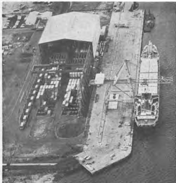
Aerial view of Port of Melbourne, one of the world's first ports to use Twin-Container Terminal Systems. Containers are handled in pairs by Twin-Lift Portainer cranes and Twin-Lift Transtainers or terminal cranes.
