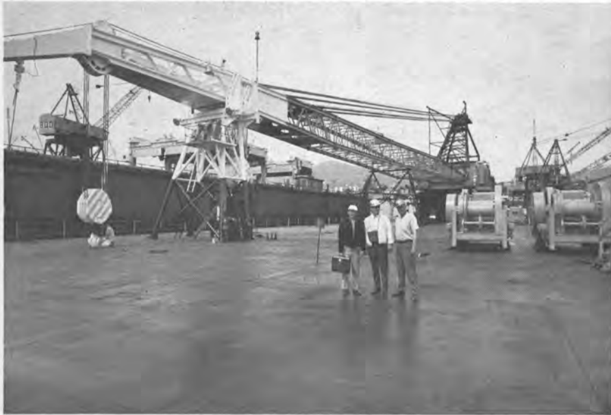
Deck view of the huge offshore construction crane barge built by Burrard Dry Dock Company Limited for Raymond International. It is 350 feet long and 100 feet wide.
