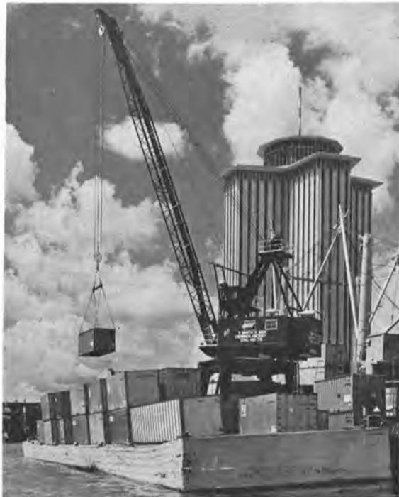
High-gantry 60-ton capacity Mickey transferring containers from a ship to a barge and loading some on its own deck.
