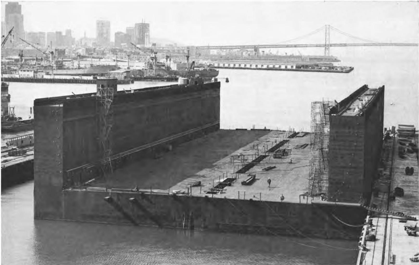
March, 1970. San Francisco's big drydock is being fabricated in quarter-sections. Here, the first two have been mated, and the half-dock unit is ready to be joined by the remaining two sections after their completion and launching. The finished dock will then be moved to its mooring basin, now being dredged at the site of the yard's old Pier Six. Bay Bridge is in background.
