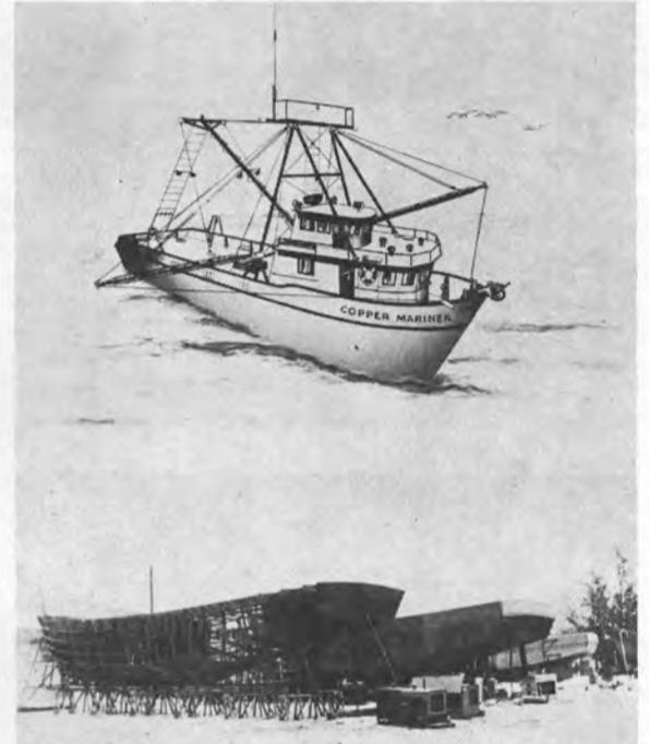
Artist's conception (top) of the Copper Mariner, copper-nickel-hulled shrimp trawler presently under construction. A four-year in-service test program will determine savings in operating and maintenance costs resulting from use of the inherently corrosion-resistant and non-fouling copper-nickel hull material. The Copper Mariner under construction (bottom) at Salina Cruz in Oaxaca, Mexico. Projected launching date is September 1970.
