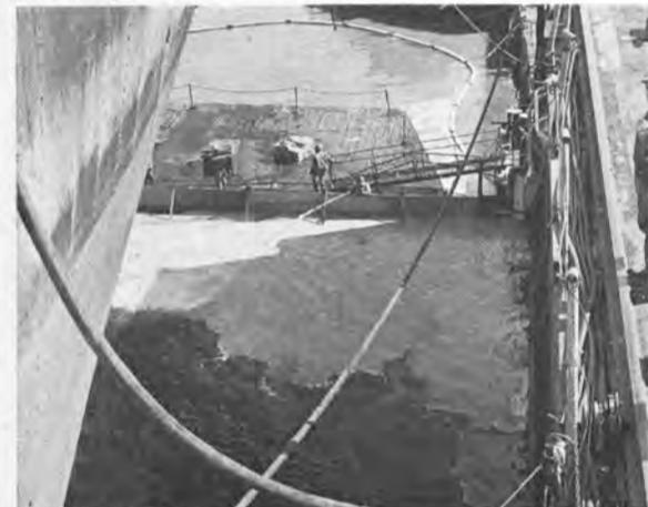
Effective use and careful monitoring of sealed barricade and slickbar floating oil boom aid the containment and removal of oil, preventing pollution of the Mississippi.
