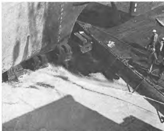
Entrapped oil from the vessel's tanks and oil water is chemically treated as it is pumped from the barricaded drydock to the disposal barge.
