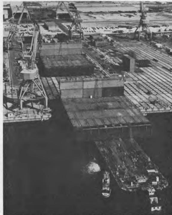
Massive launch pontoon sections move forward on rails from the construction site to the launching barge in the Pascagoula channel.
