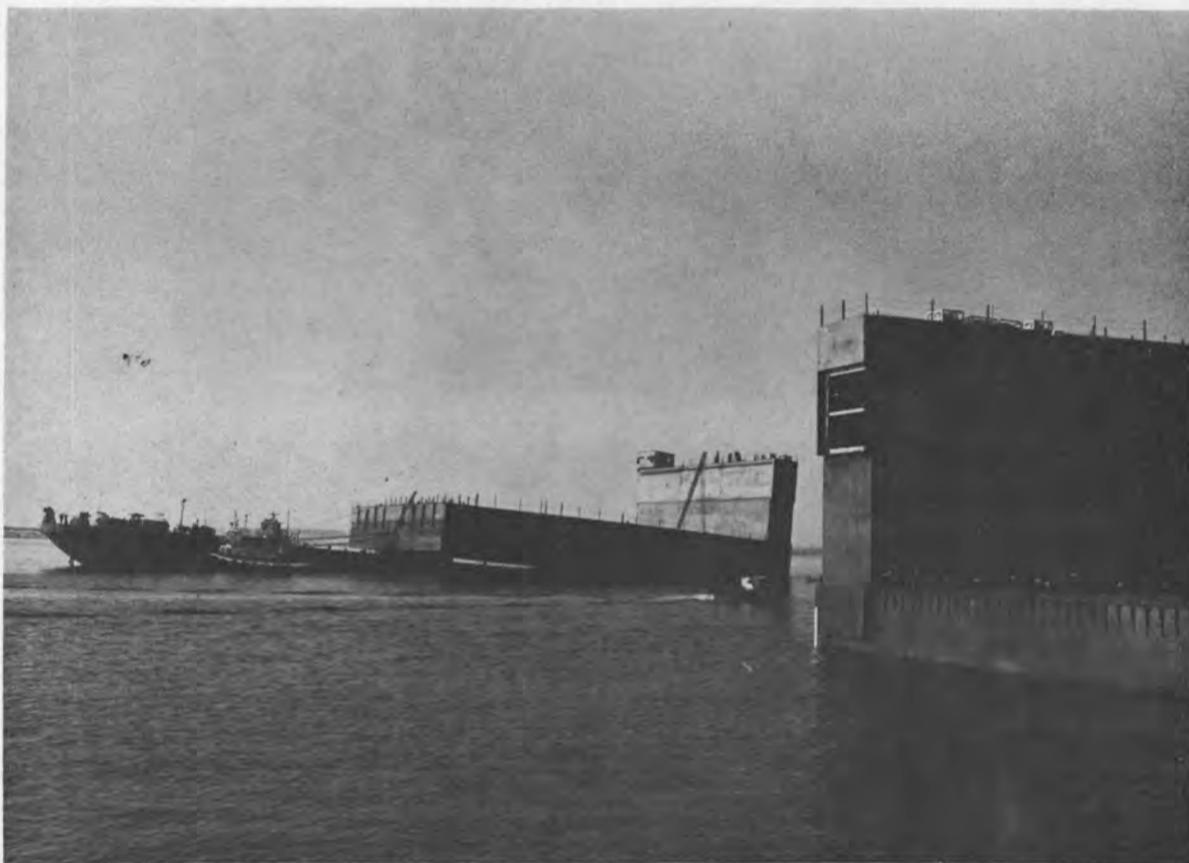
**ON THE COVER:** One section of the unusual pontoon launch, minus the removable wing, slides from the partly submerged barge in midstream as another section floats free in the foreground 500 yards from the assembly area.
