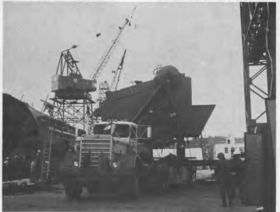
The first of two B&W boilers for the Doctor Lykes is moved into position for lifting aboard the vessel at the Quincy Division shipyard of General Dynamics in Quincy, Mass.
