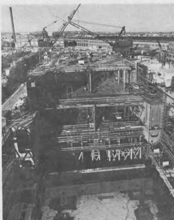
This stern view shows the cantilever sections extending beyond the stern. In the foreground are the first two girders for the elevator platform.
