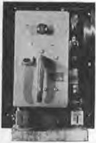
Westinghouse DAN-30 air circuit breakers — 250 volts—500 amps DC—with reverse current overload trip units. Built for 60 KW—120 volt DC machines.
