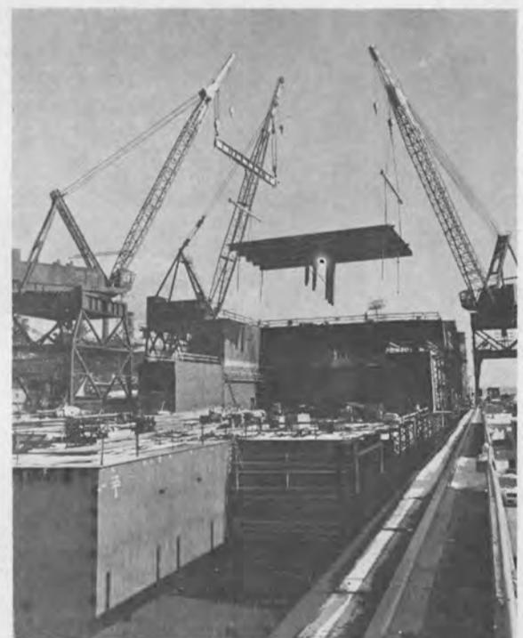
Landing a 95-ton upper deck section on the Doctor Lykes on January 20 brought the steel erection to over 50 percent completion for the first ship.
