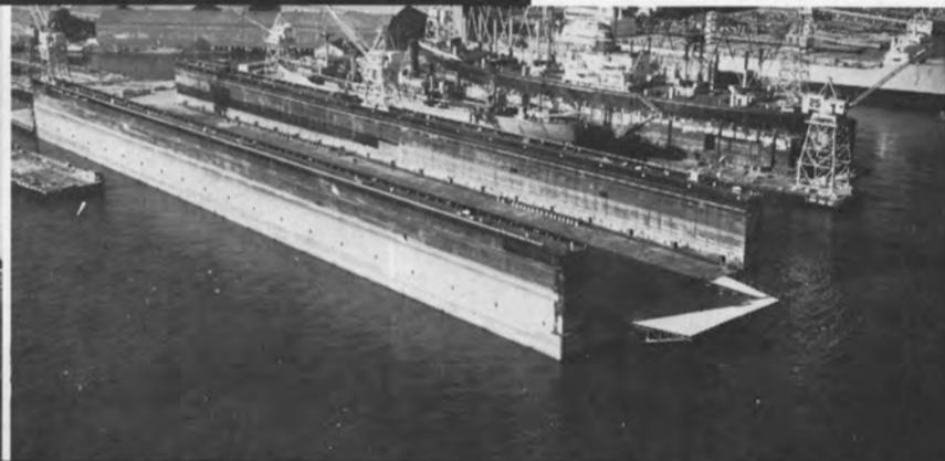
New dock can lift 65,000 tons and accept a vessel of max 150-ft beam and 31-ft draft. Pontoon is 20 ft deep, has 800-ft-long unobstructed deck—plus two 50-ft, grate-type aprons. Its 2,000 pumping hp can lower and raise the unloaded dock in less than 40 minutes.
