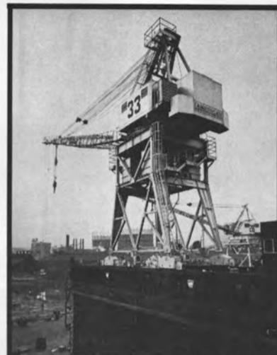
Each wingwall carries a 60-ton crane with 90-ft boom. Centerline lift with spreader bar: 120 tons.
