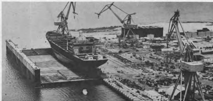
2. In this view the ship has been moved onto the launching platform. This transfer from shore to platform is by means of a special wheel-on-rail transfer system. The total transfer distance is about 300 feet and required four hours to complete, as the ship was moved at a rate of 22 inches a minute. The platform can support 57,000 tons.
