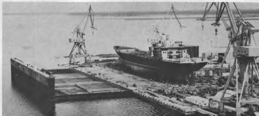
1. The Austral Envoy prior to launching on the shipyard's integration area where the various modules of the ship were joined together to form the completed hull.
