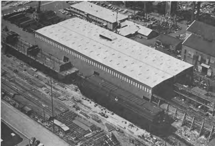
Tidewater Barge Lines, Inc.'s Barge 44 (lower right) undergoes final launch preparations at the Marine Construction Division of Zidell Explorations, Inc. The 3,000-ton-capacity barge is fifth of identical series placed in service by Tidewater.
