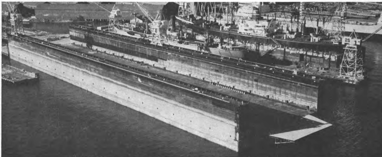
The nation's largest floating drydock was placed in service in 1970 at our San Francisco ship repair yard. Measuring 900 ft over the aprons by 150 ft between wingwalls, it will handle most ships up to 150,000 dwt—and some as large as 230,000 dwt.
