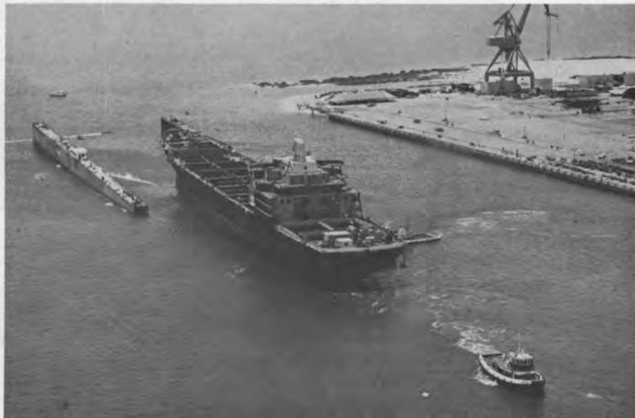
4. The launching platform with the ship is moved into the middle of the ship channel by means of a special out-haul system utilizing two self-contained mooring winches and two spring-line winches. The dock is ballasted by 48 pumps, powered by on-board generating equipment, and the ship is floated off the platform. The traditional bottle of champagne is broken at this time by means of electronically operated release activated by the sponsor. The reverse process can be used to dry dock a ship.
