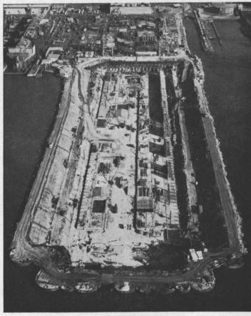
The nation's largest building basin is nearing completion at our Sparrows Point Yard. Measuring 1,200 by 200 ft, it can accommodate the construction of ships as large as 300,000 dwt. A new panel shop and a new abrasive-blasting and paint building (behind the basin) have already been completed.
