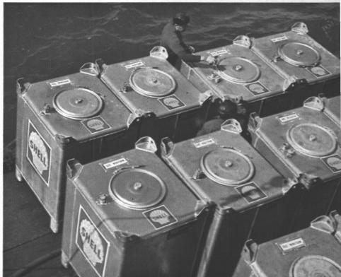
"Jumbo tanks" positioned on lighter of Standard Boat Company. Each jumbo is "dedicated"—receives only one type of oil—thus assuring freedom from contamination.
