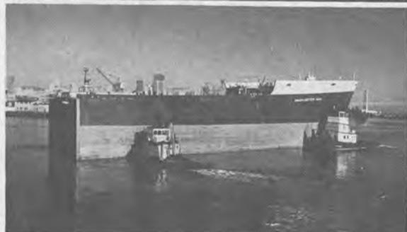
The new 105-foot long mid-body section (top) is shown being floated into position during the conversion. This exacting maneuver occurred after the vessel had been cut in two and the bow section floated out into San Francisco Bay (bottom).
