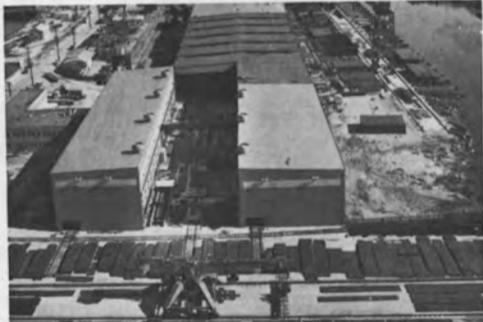
Fabricating shop was lengthened by nearly 600 ft and a roll shop added. Plate handling has been improved by the new electric hammerhead crane (foreground and above) and by electric transfer cars which bring stock from the storage yard into the shop.
