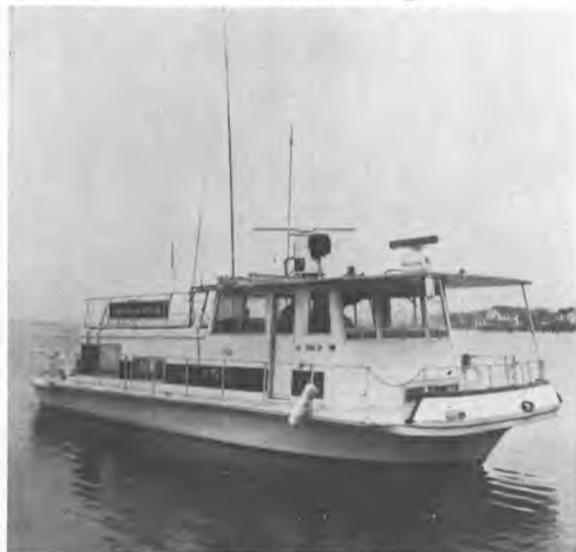
The converted 43-foot houseboat is outfitted with more than \$50,000 worth of new radar systems and other communications and navigation aids made at Radiomarine's Red Bank, N.J. plant.
