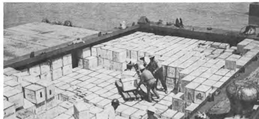
A LASH lighter stowed out 100 percent with a cargo of tea. Rapid discharge and loading rates are possible by the easy vertical load stow design conditions of the lighter. The cargo is worked from the top down for effective and safe stevedoring operations.
