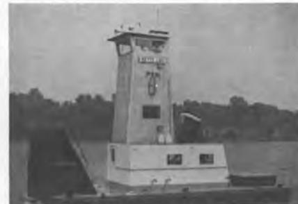
Aluminum tower on the Betty Lou affords the operator a 24-foot-high eye level for safe navigation when pushing high barges.
