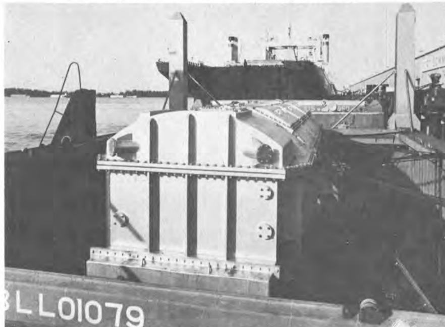
Seen in the foreground is one of the heavy lifts which was in excess of 255 long tons. Portable extension posts are shown fitted to the LASH lighter lifting posts which allow for the transport of lifts under deck up to 22 feet in height.
