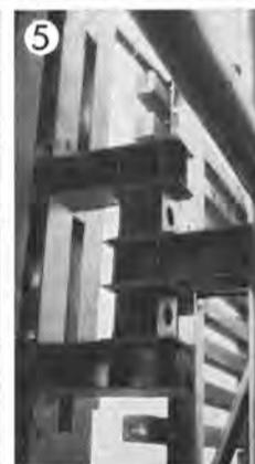
(5) And our new Shear-Type Dock Fenders, which can absorb a remarkable 200% deflection load without a groan.
