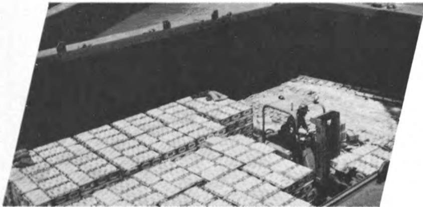
Fork lift discharges LASH barge load of beer in palletized Shrink-Paks.
