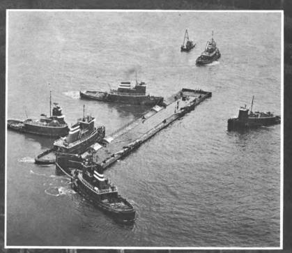
bed. Right where sandhogs could link it to tunnel sections previously hewn through Welfare Island's bedrock.
