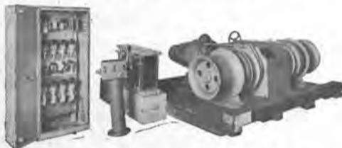
For 1-5/16" chain—on 36" centers. 15 H.P.—115 volts DC—1750 R.P.M.—6000 lb. line pull.
