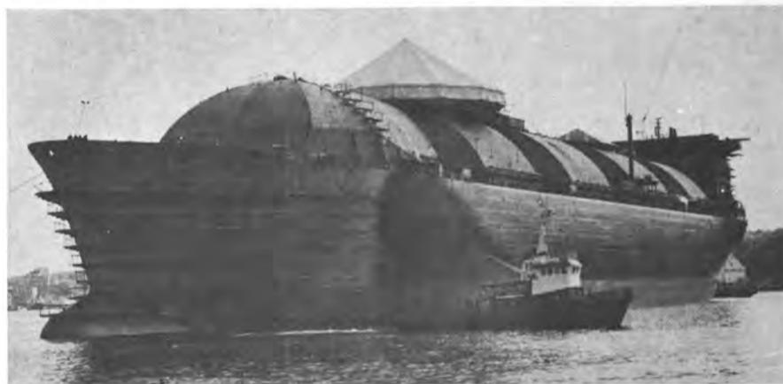
**THE NORMAN LADY** under control of tugboats immediately after launching at the Rosenberg Verft in Stavanger, Norway. The tank covers and erection tent provide a unique profile.
