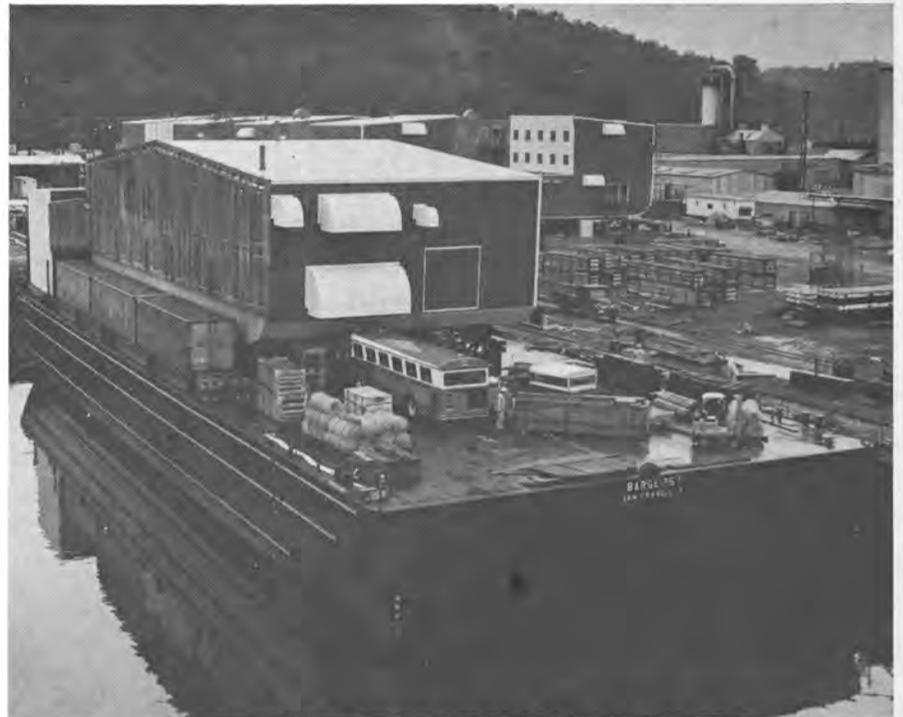
Shown on a barge is one of five sections of the B.P. Alaska, Inc. base operations camp that will be carried to Alaska's North Slope. In the background are four sections of the camp yet to be loaded.
