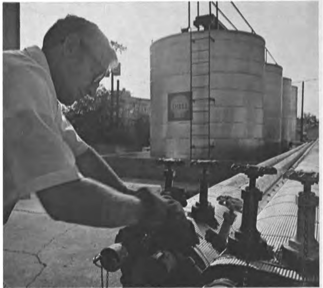
E. J. Wheeler, Manager of Marine Oil Services, Inc., opens an outlet valve so that ALEXIA Oil can be pumped at 55 gals./minute into a waiting tank boat. Four insulated 10,000 gallon storage tanks hold Shell lubricants at a constant 120°F., permitting fast flow in any season.
