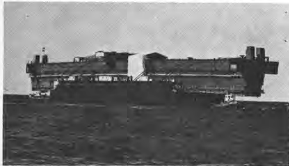
The 607-foot girder hung over both ends of a floating dock for the trip from Copenhagen to Malmoe.
