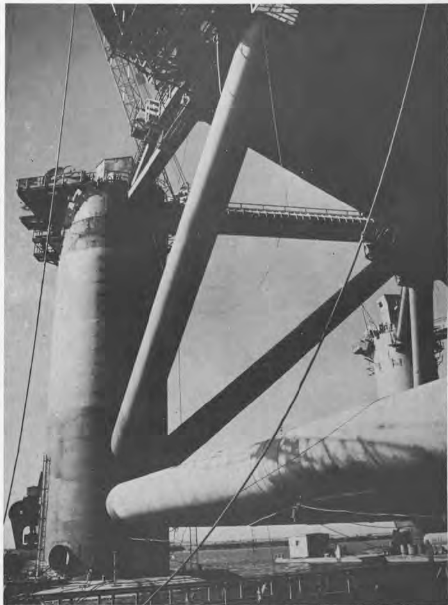
ONE OF FIVE —Each of the columns has a diameter of 31 feet 4 inches and a pontoon at the foot measuring 70 feet in diameter and 23 feet in height. It is 134 feet from the base of the pontoons to the main deck. The draft when under tow is 24 feet and during drilling operations the draft is 72 feet. The horizontal bracing tubes have a diameter of 8 \frac{1}{2} feet and a diagonal of 7 \frac{1}{4} feet. The platform forms the upper tie.
