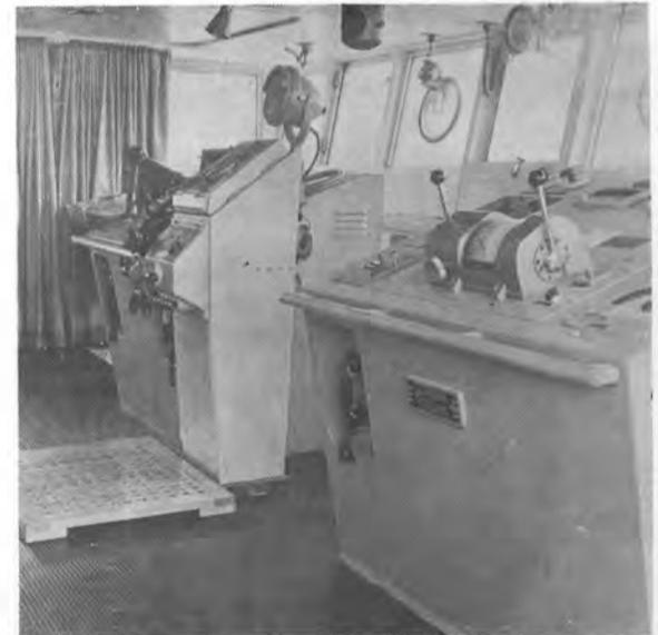
Looking to the port side of the bridge shows the propulsion control console, navigating units and the radar.
