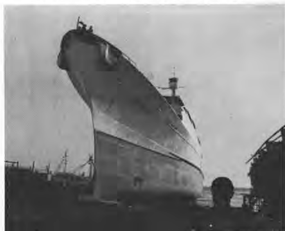
Sliding down the ways into San Diego Bay is the Sandra C., newest 1,200-ton-capacity tuna superseiner. Shown under construction at the right is her sister ship, which will be named the Marjorie R.
