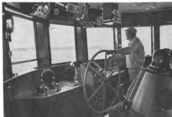
Pilothouse, showing steering station and control console.
