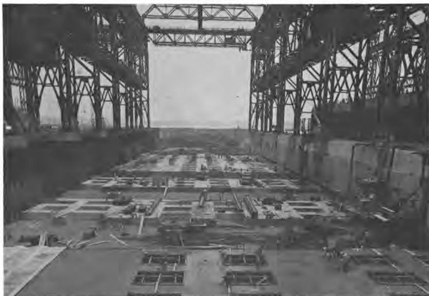
Workmen are nearing completion of the concrete slab floor on Building Basin Twelve at General Dynamics, Quincy Shipbuilding Division. The Basin will be the site of the first liquefied natural gas tanker to be constructed in the United States.
