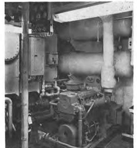
Detroit Diesels drive the Delco generators for electric power.
