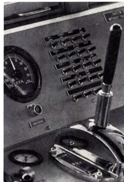
main control panel
