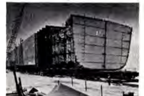
Catug construction seen from bow portion
