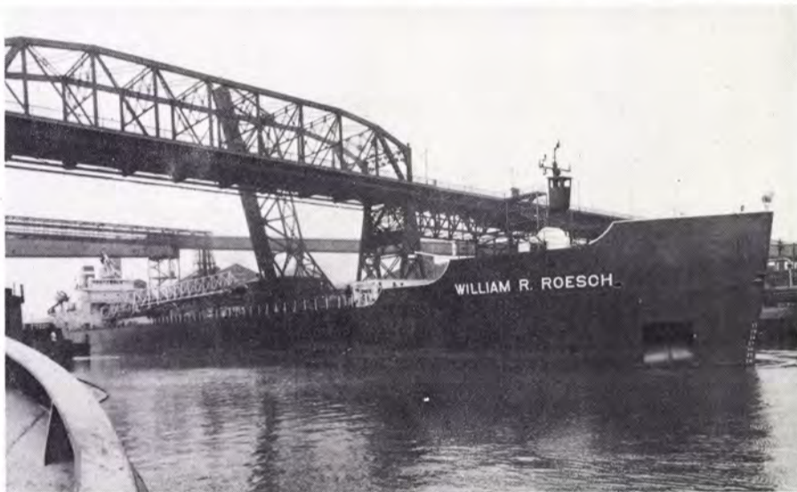
NEW GREAT LAKES ORE CARRIER, M/V WILLIAM R. ROESCH is Power Bossed by two ALCO, V-16, 251 diesels rated at 2800 BHP each.
