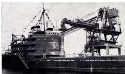
Bulk Loaders —This bulk loader, operated by one man, handles 750 Long Tons per hour of Alumina; 1000 Long Tons per hour of Bauxite. Designed with slewing upper tower and hinged apron.
