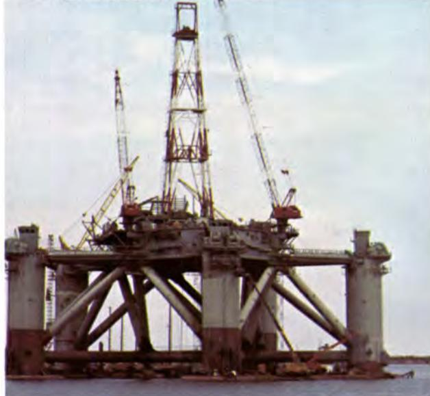
**CLYDEBANK, SCOTLAND** *Penrod 64*, jackup, hull dimensions of 230' x 200' x 26'; 6,000 tons. Designed for TD of 30,000'. Crew of 78. Scheduled to operate in North Sea.
