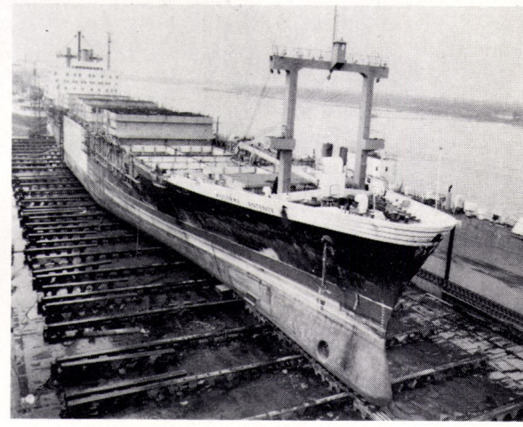
The Farrell Lines containership S/S Austral Entente shown in drydock at Avondale Shipyards in New Orleans after new 144-foot midbody was added to bring the vessel's overall length to 813 feet and effectively double its refrigerated cargo-carrying capacity.
