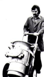
The Jetfan 125 is truly portable, weighing only 43kg (95lbs) it can be easily installed, converted, and operated by just one man.
