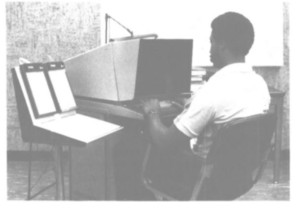
A computer drafter sits at the console of one of five computer graphics modules in the Computer Graphics Section at Marathon Marine Engineering Company, on which a drafter-operator can draft a design for an offshore jackup drilling rig twice as fast as by the manual procedure.
