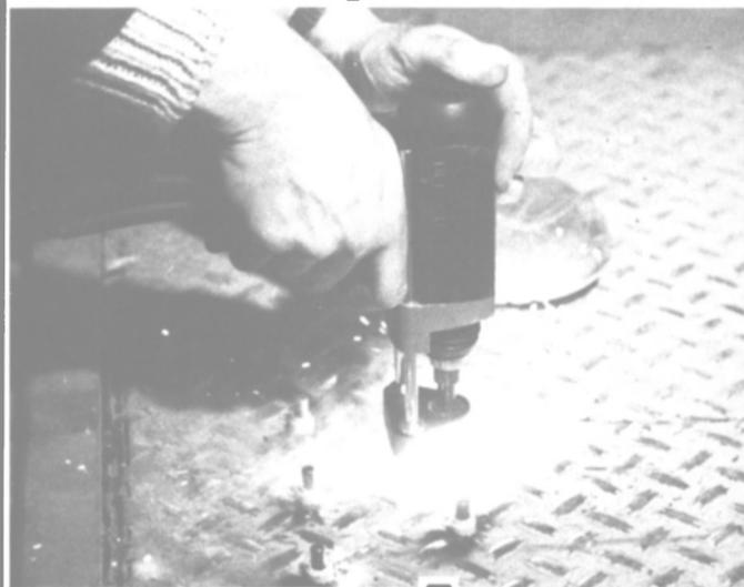
■ Nelson® studs are small steel projections that may be welded
