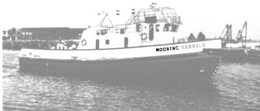
New mooring tug *Mooring Service*, built by Halter for Zapata Marine Service, has collapsible mast to facilitate line handling.
