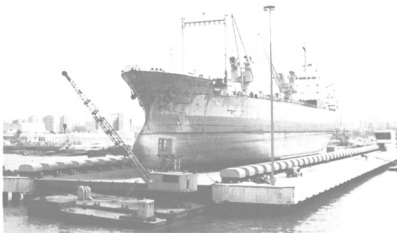
Water level view of 25,000 DWT vessel on platform.
