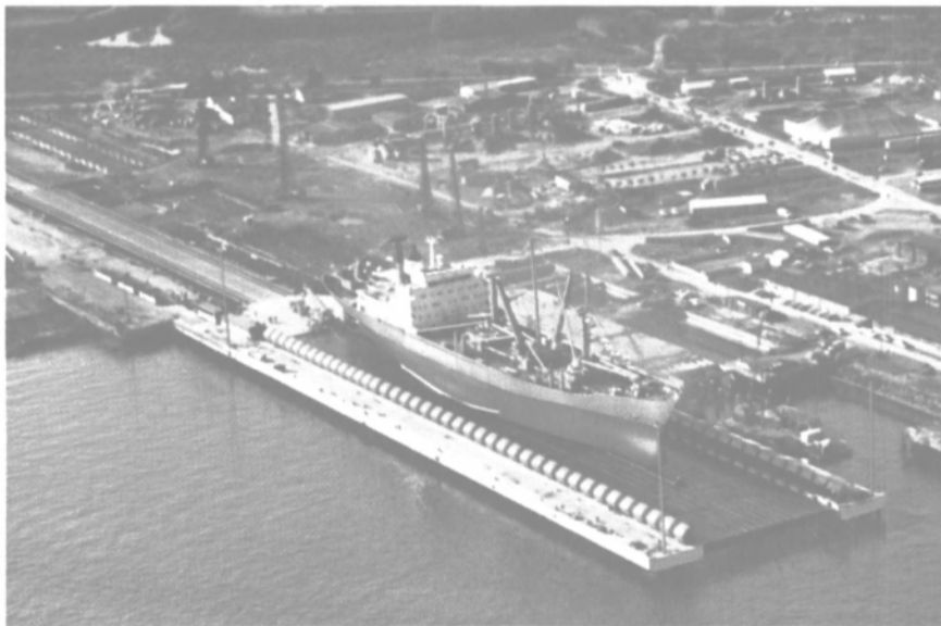
25,000 DWT vessel on platform awaiting transfer.
