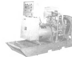
100 KW 440/220/3/60 generator driven by GM 4-71-T radiator cooled turbo charged diesel. P.F. 0.80—for T-2, etc. 1800 RPM. With switchgear. Generator is 10 wire—all voltages possible.
