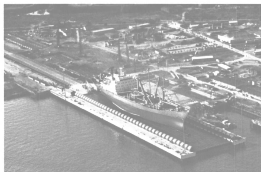
25,000 DWT vessel on platform awaiting transfer.
