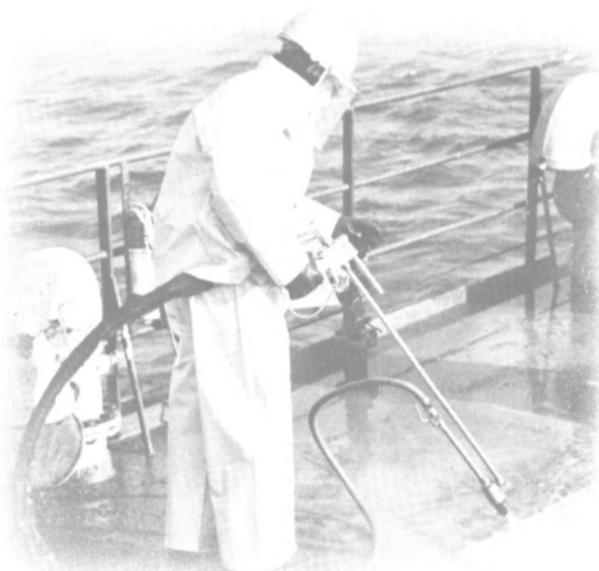
poop deck. The job was done as routine maintenance with interruptions for bad weather and all-hands tasks. In a little over two weeks the poop deck was "white-metal" cleaned and freshly painted.
