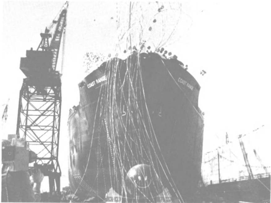
Products carrier *Coast Range* sliding down the ways after recent christening at National Steel and Shipbuilding yard in San Diego. Powered by 13,000-shp General Electric steam turbine, the 37,500-dwt vessel is for Union Oil Company of California. She is second of three sisters.
