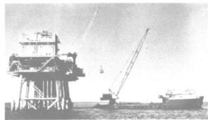
The Lift Tide (shown above), a derrick/ supply vessel operated by Tidewater Contractors, Inc., a subsidiary of Tidewater Inc., is now in U.S. Gulf service off the Louisiana coast following extended duty in the Middle East. Refitted with a new American Hoist & Derrick, Model 9760, 90-ton lifting capacity, pedestal-mounted crane, the vessel is certified by the U.S. Coast Guard for unrestricted ocean service.
