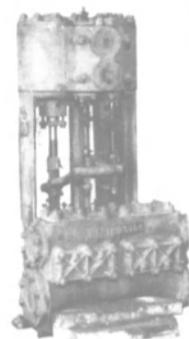
Ex-T2 Tanker. 150 Lbs steam—10 in exhaust — 100 lb discharge. 6" suction — 4" discharge — 1½" steam — 2" exhaust. Overall ht 4'7½" — OAW 3' — Depth 2' 9".
