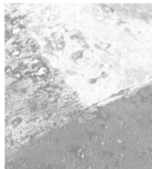
Heavily rusted deck (below), after water blasting (left), and "white-metal clean after water-sand blasting (right)."
