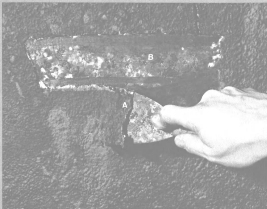
Photo from ABSTECH report shows no rust damage after 9½ years. When Fluid Film (A) was scraped away from ballast tanks, no oxidation was found on base metal (B).
