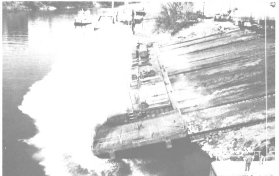
Side-launching of one of two NABRICO-built bunkering barges produced this big splash. Barges will be used by John W. Stone Oil Distributor, Inc. to refuel ships and towboats in the New Orleans area.
