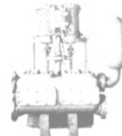
10 X 11 X 12 — Worthington — 560 GPM @ 125# G. 8" Suction — 6" discharge pumps bronze fitted.
