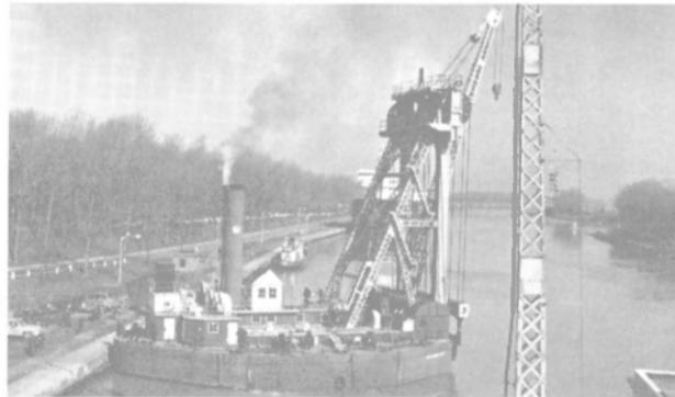
1. Gate lifter, 500 ton lifting capacity, electrically controlled, c/w upright steam boiler, 160 lbs. steam pressure capacity. Engine: W.H. Allen & Sons 290 BHP 400 RPM, 10" stroke, 12 1/2"x22" cylinder. Generator: 200 K.W. 240 volts, 833 amps, 400 RPM. Mounted on Moulded Hull Barge, 62' wide, 90' long, 26' deep, 15' draft, overall height water line to top of boom 120'.
