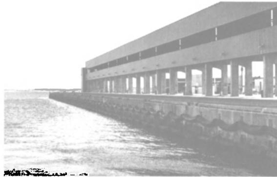
A double row of several heavy duty tubular rubber fenders are fastened in place with chains letting each section independently perform protection to both vessel and dock.
