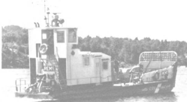
2. Landing Craft, M.V. Remy, built 1943. Powered by two G.M. Diesels, 175 H.P., 52' long, 14' wide, 4'6" draft, c/w McDougall Water Pump with Briggs and Stratton Engine, 4 cycle, 1 cylinder, 3 H.P.
