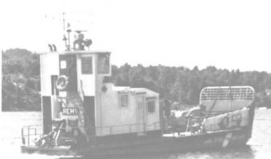
2 Landing Craft, M.V. Remy, built 1943. Powered by two G.M. Diesels, 175 H.P., 52" long, 14' wide, 4'6" draft, c/w McDougall Water Pump with Briggs and Stratton Engine, 4 cycle, 1 cylinder, 3 H.P.
