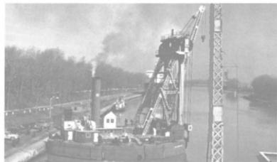
1 Gate lifter, 500 ton lifting capacity, electrically controlled, c/w upright steam boiler, 160 lbs. steam pressure capacity. Engine W.H. Allen & Sons 290 BHP 400 RPM, 10" stroke, 12½"x22" cylinder. Generator 200 K.W. 240 volts, 833 amps, 400 RPM. Mounted on Moulded Hull Barge, 62' wide, 90' long, 26' deep, 15' draft, overall height water line to top of boom 120'.
