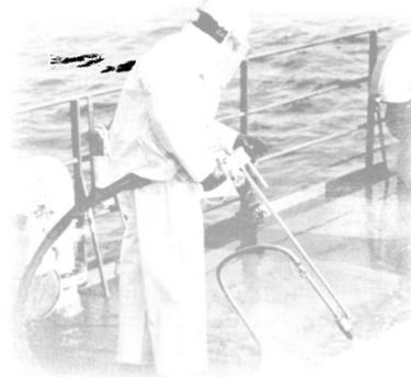
poop deck. The job was done as routine maintenance with interruptions for bad weather and all-hands tasks. In a little over two weeks the poop deck was "white-metal" cleaned and freshly painted.
