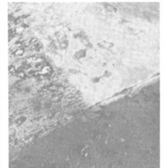
Heavily rusted deck (below), after water blasting (left), and "white-metal clean after water-sand blasting (right)."
