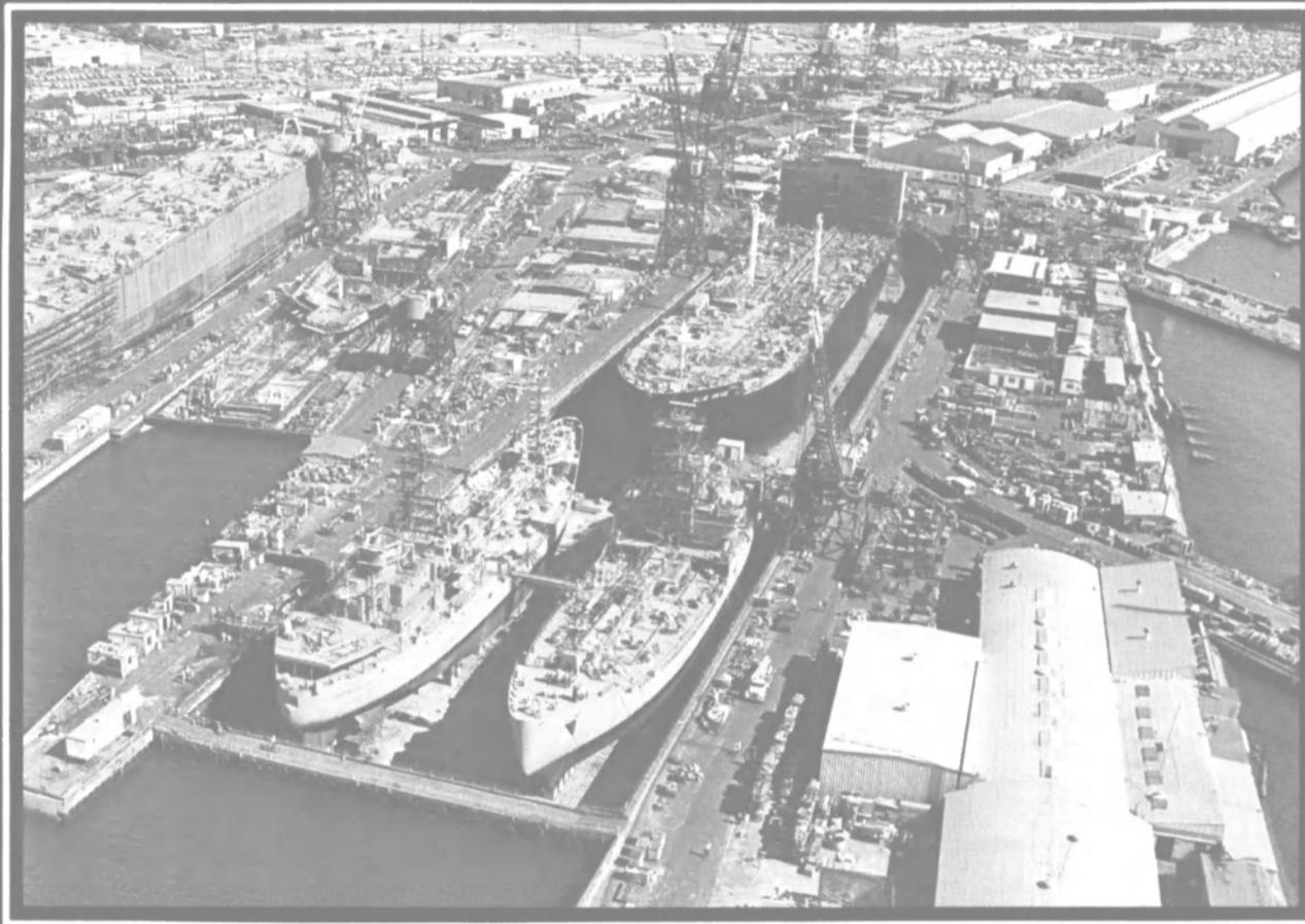
NASSCO's 1000' x 175' graving dock being fully utilized to build the first of three 37,500 DWT Carlsbad Class Product Tankers for Union Oil and to reactivate/re-engine two Alatna Class T-AOG gasoline tankers for the U.S. Navy (MSC).
