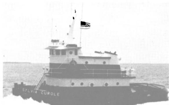
Patti Industries recently delivered the 65-foot Sylvania Curole to T.U. Gruidry and Reynolds Curole. The 1,000-hp tug is powered by GM 12V71 engines.
