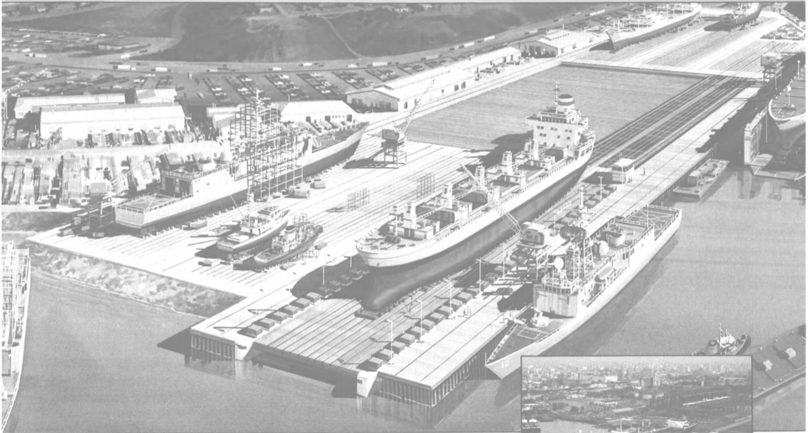
Todd Pacific Shipyards Corp., Los Angeles division, has just become the newest member of the Syncrolift family . . . now 148 installations in 58 countries. When completed, the Todd Syncrolift will be the largest shiplift in the world . . . 655 feet long, 106 feet wide, with a lifting capacity for vessels up to 48,000 DWT. An adjacent transfer system will enable the yard to service five maximum size ships ashore at one time.
