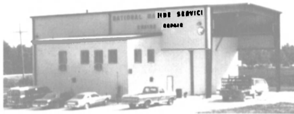
The new engine repair shop at the National Marine Service Canal Yard in Harvey, La.
