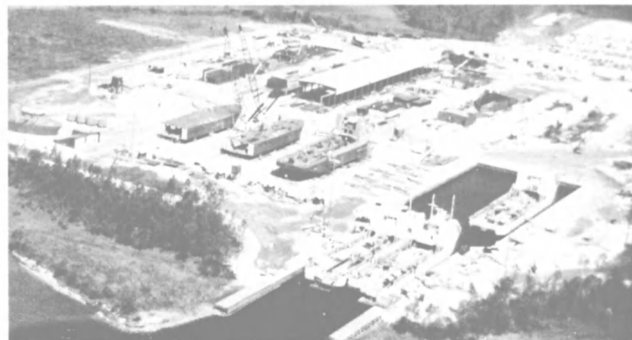
View of Eastern's Allanton yard, which was opened in 1981, showing Seahorse boats under construction.
