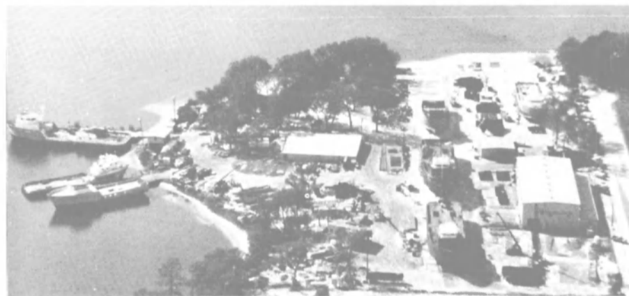
Vessels under construction at Eastern Marine's yard at Panama City, Fla.
