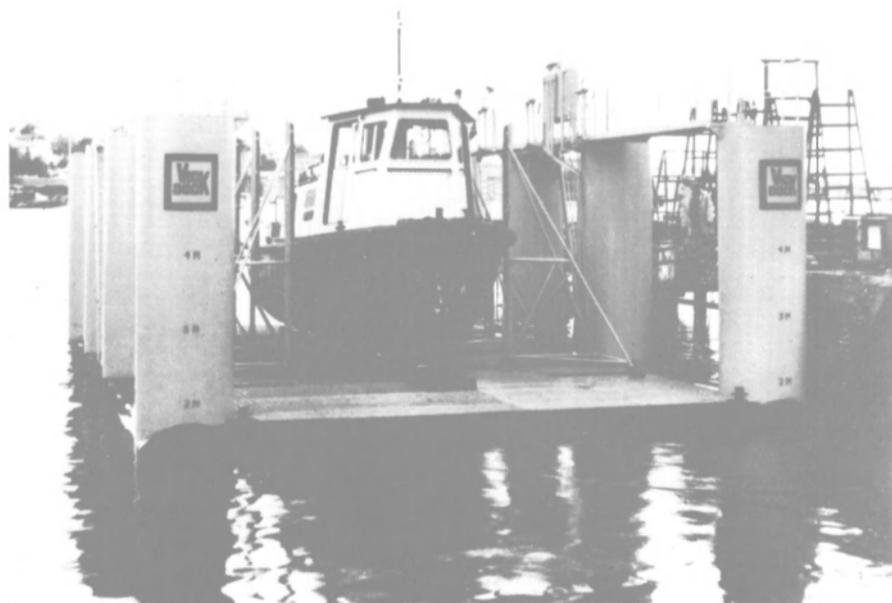
Unique floating drydock that uses compressed air to blow water from its ballast tanks will be built by companies in the U.S. and Canada.
