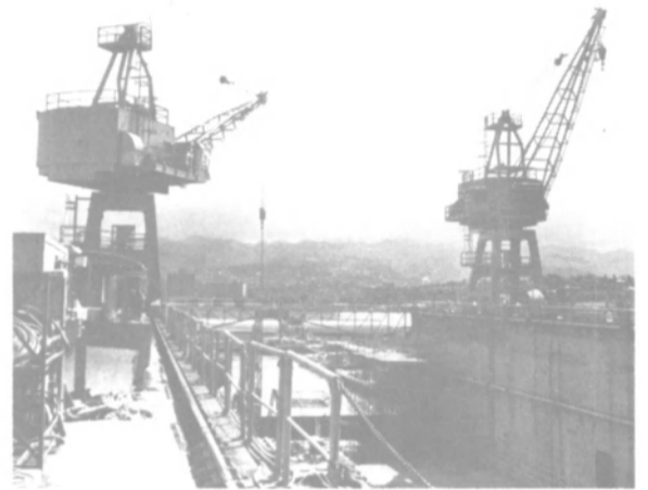
New type diesel-electric cranes have been installed on Navy's floating drydock USS Competent at Pearl Harbor.
