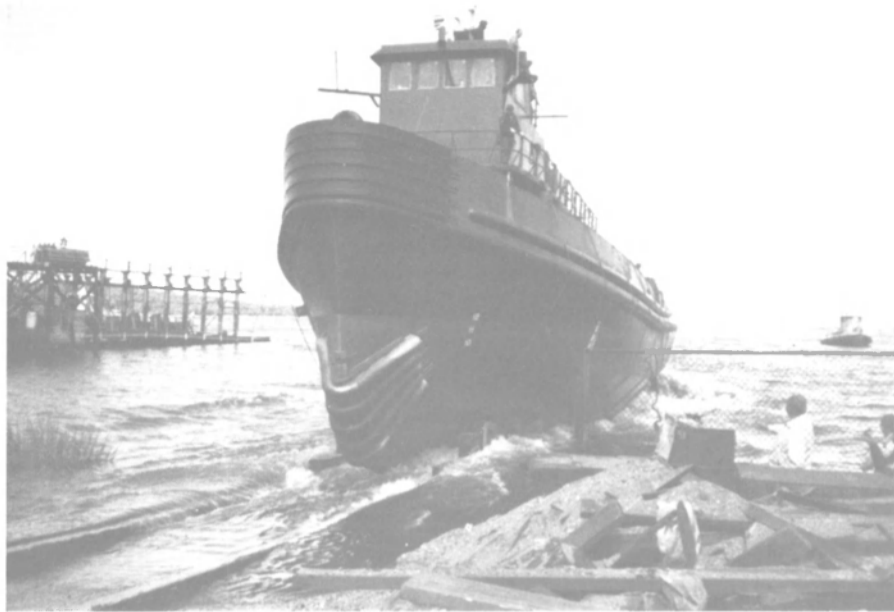
EMD-powered twin screw tug Chessie sliding down the ways at Jacobson Shipyard.
