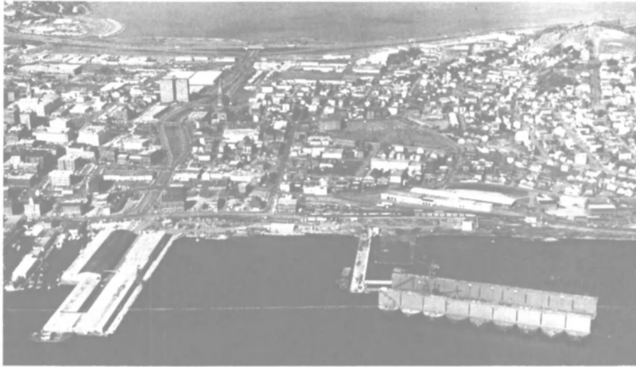
New repair facility operated by Bath Iron Works in Portland, Maine, features 81,000-ton drydock shown at right. Old Maine State Pier at left has been converted into modern repair shops, warehouses, and offices.
