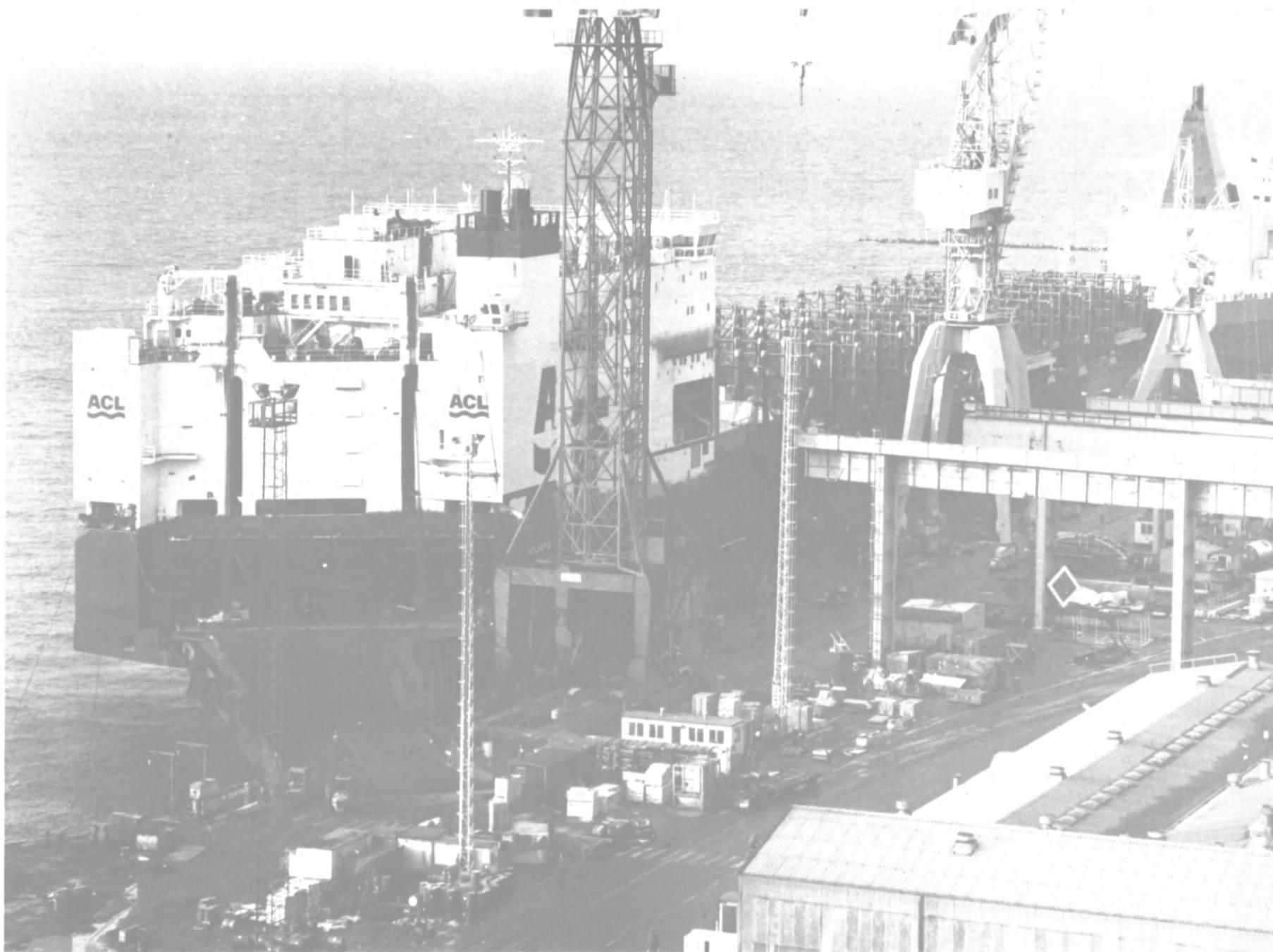
Atlantic Container Line's RO/RO-container-ship **Atlantic Companion**, first of five that will enter service this year, is the largest and most technologically advanced vessel ever built for the North Atlantic trade. The Kockums-built ship has a capacity for 2,130 TEUs as well as space for 600 automobiles. Major features include the huge stern ramp and permanent cell guides on the weather deck, both supplied by MacGregor-Navire.
