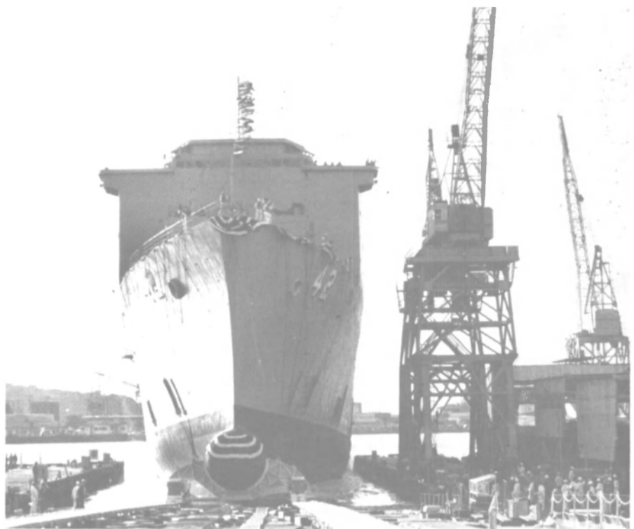
U.S. Navy Dock Landing Ship Germantown (LSD-42) splashes into Seattle's Duwamish River after being launched by Lockheed Shipbuilding Company's inclined shipway.
