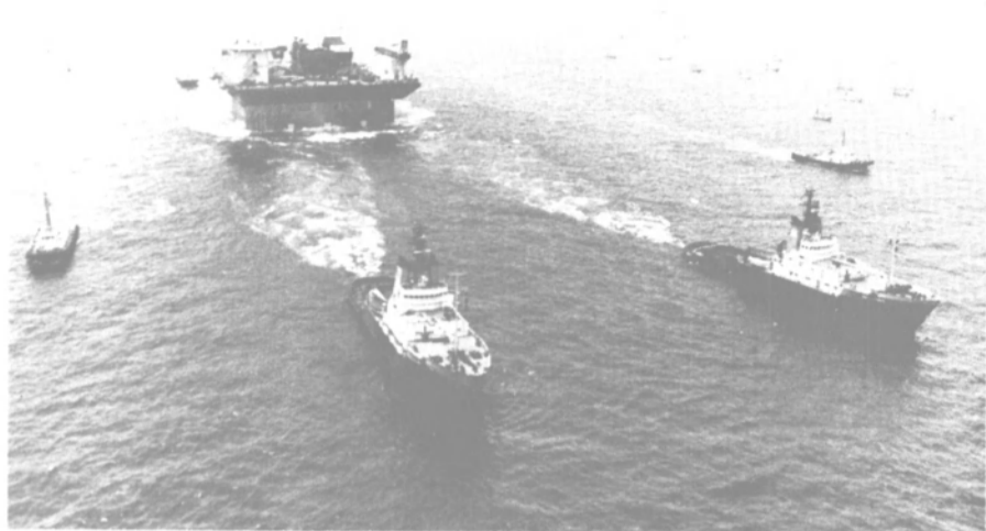
The tugs Smit Rotterdam and Smit London towing the Concrete Island Drilling System.
