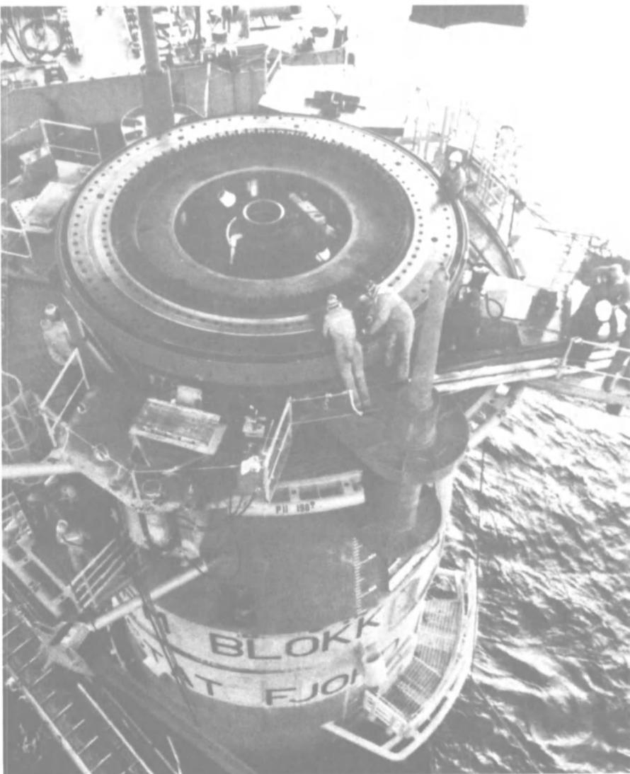
Rotating superstructure of ALP is joined to riser column by 640-mm-diameter double roller bearing. Column attaches to anchor base via a 200-ton universal joint.
